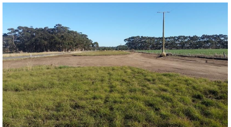
Topsoil removal to a depth of approx. 100 mm from sections previously dominated by exotic species. These areas will be sown with a diverse native grassland seed mix to reconnect the preserved areas of Plains Grassland (foreground and background).
